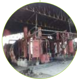
Tyre Pyrolysis Plant Ratlam, Madhya Pradesh
